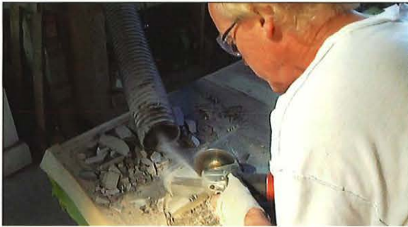
While grinding stone, a worker uses local exhaust ventilation to remove silica dust and reduce his exposure.
