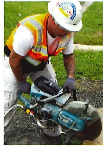
Applying water to the blade of a handheld power saw reduces the amount of dust created when cutting.
